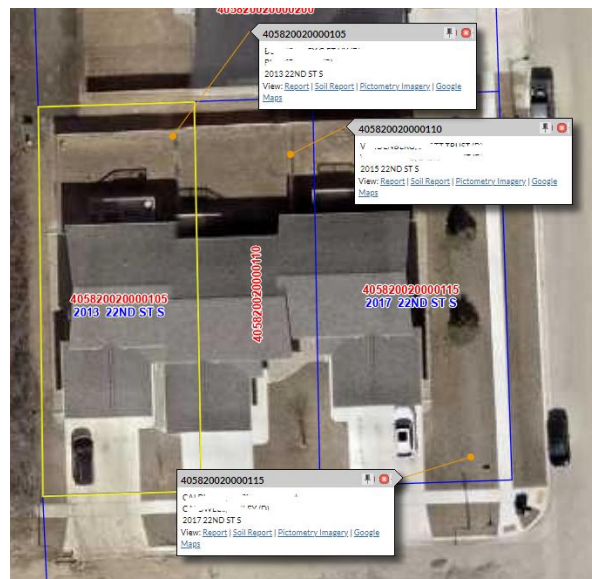
Figure 5 – Example of Zero-Foot Side Yard Structure Dwelling
